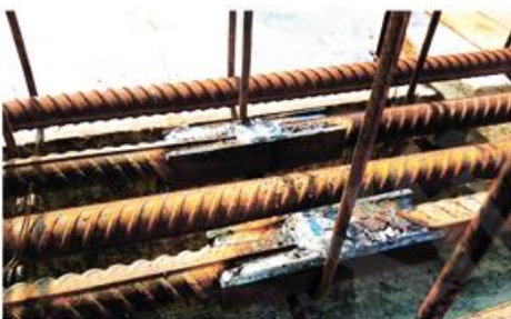
Welding connection of reinforcement for concrete
