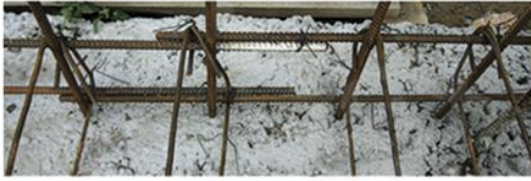
Overlapping reinforcement connection for concrete
