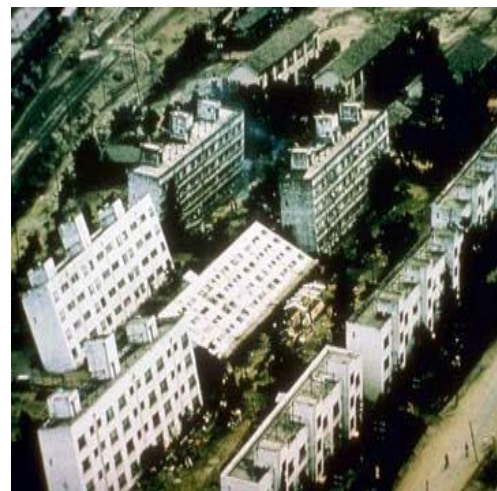
Fig 4: Some effects of liquefaction during the 1964 Niigata, Japan earthquake.
