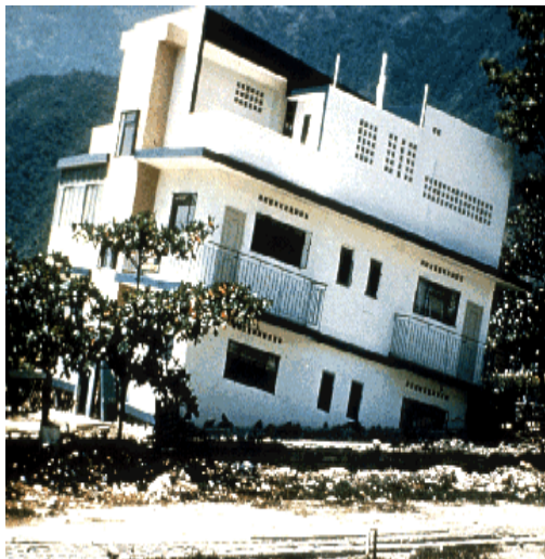
Fig 4: Some effects of liquefaction during the 1964 Niigata, Japan earthquake.
