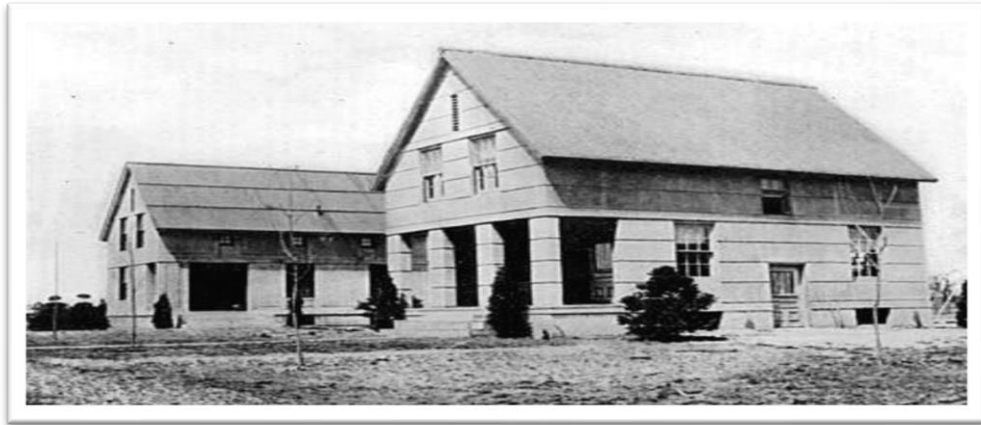
Fig. 1. One of G. Atterbury's experimental concrete houses in Sewaren, N.J. Photo by Standardized Housing Corporation / The Manufacture of Standardized Houses
