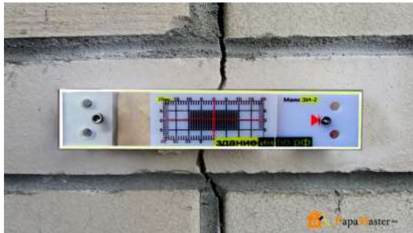
Figure 3. The process of observing cracks using beacons.
